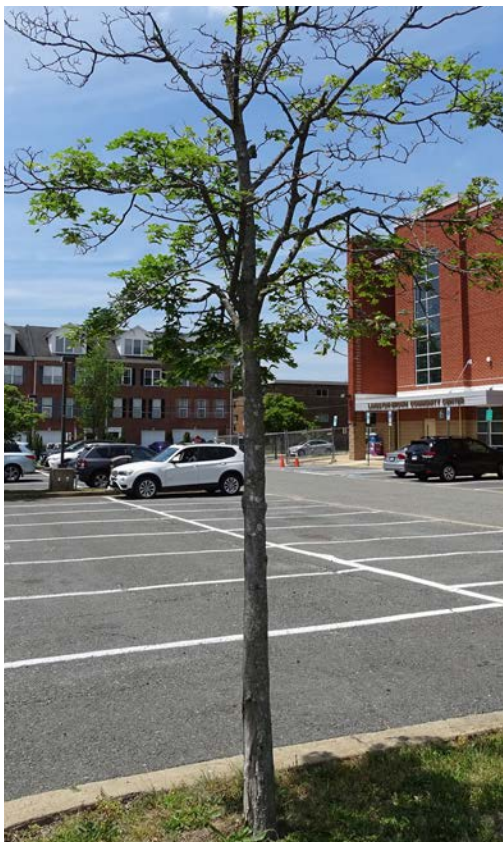
The County should remove dead and dying trees from public parking lots and consider whether the underground pit area is large enough to support new trees, whether soil volume needs to be increased, or if structural root supports are needed.
